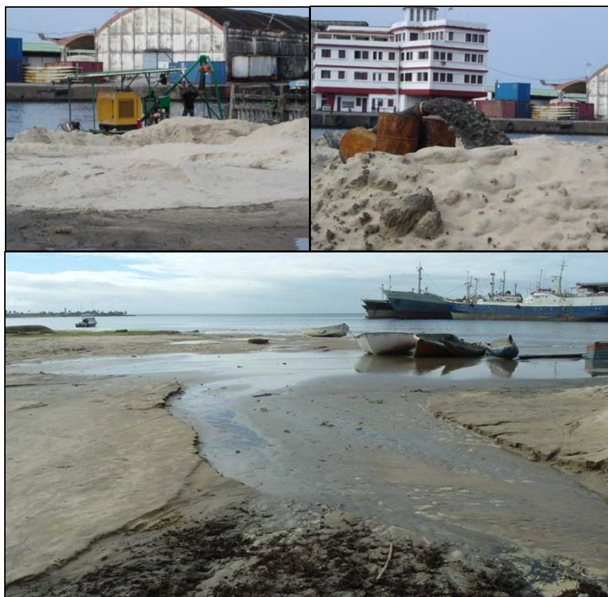
Photo Plate 3.4: The dredging operation which occurs to maintain the channel for Mole A. Spoil is pumped onto the beach and decant water returns to harbour.
