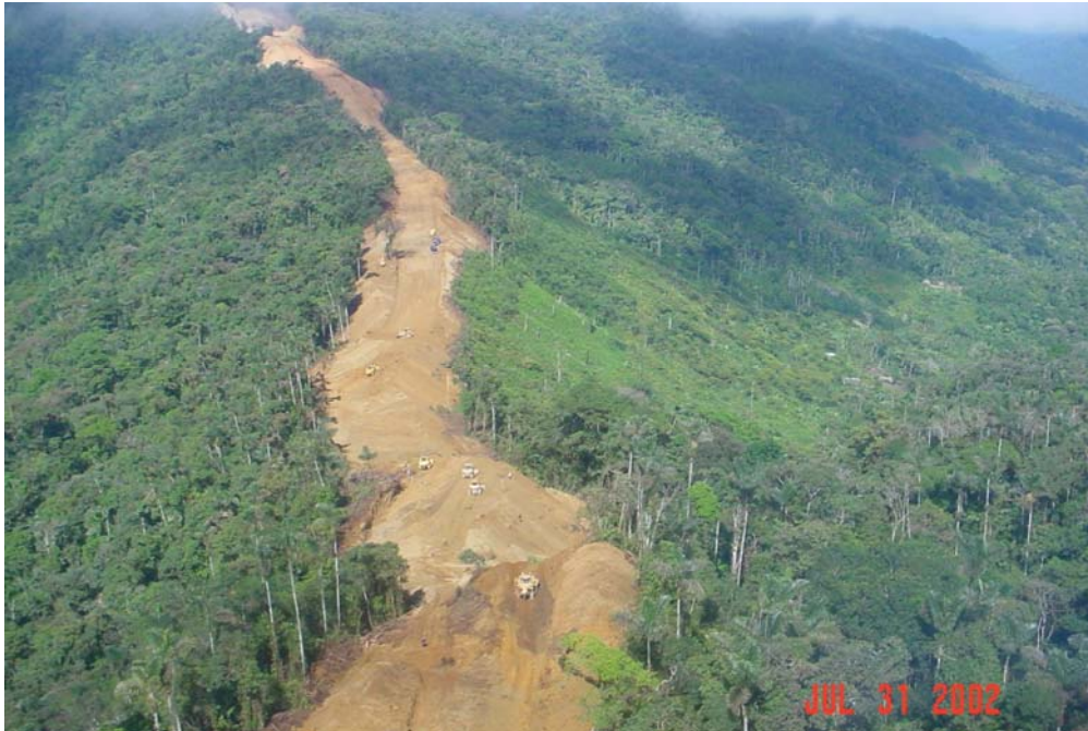
Photograph 2-1 Typical Pipeline Rights-of-Way During Construction in a Tropical Environment
