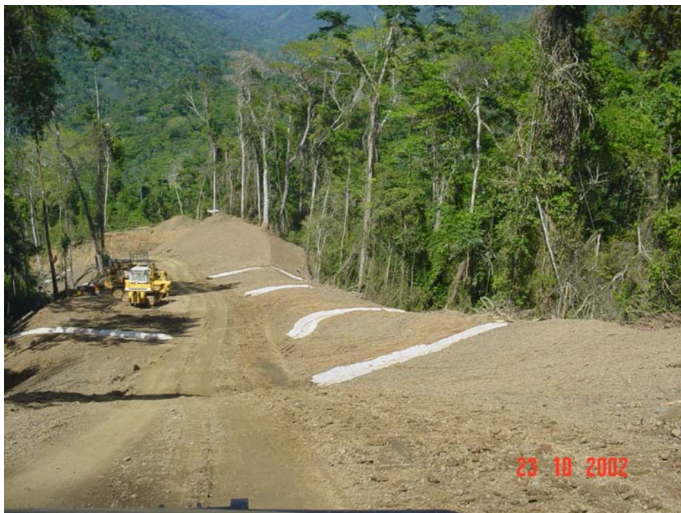
Photograph 2-2 Erosion Control on Pipeline Right-of-Way in a Tropical Environment
