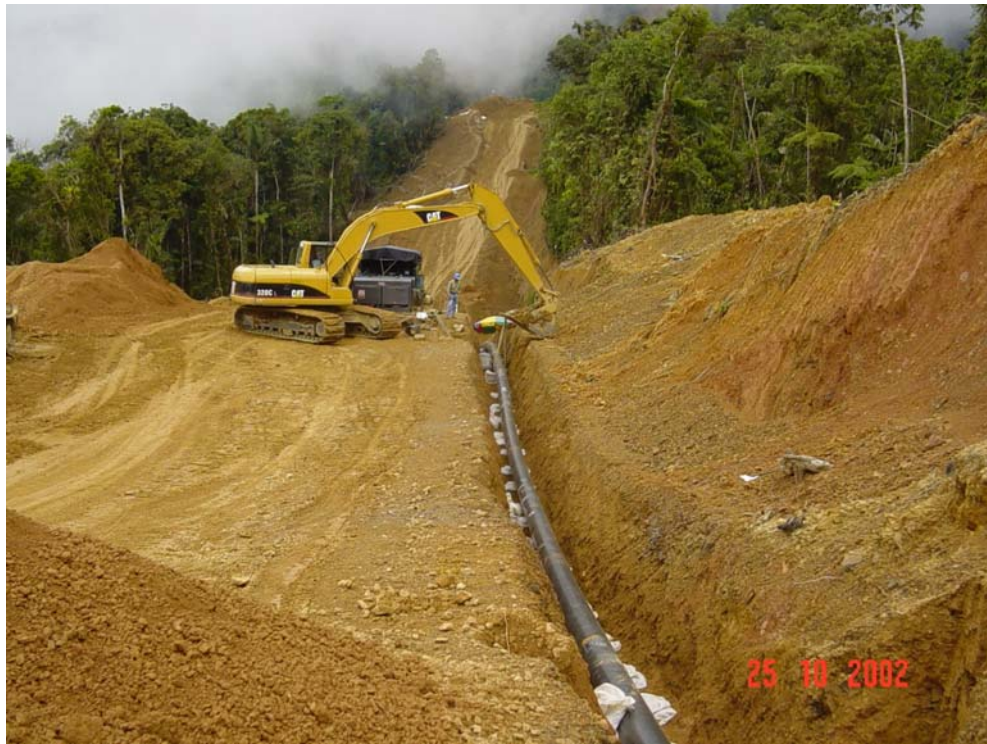
Photograph 2-3 Typical Backfilling for a Buried Pipeline in a Tropical Environment
