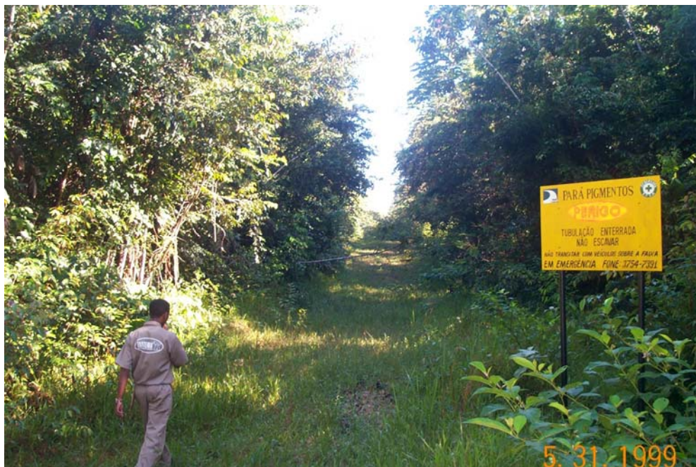
Photograph 2-4 Typical Reclaimed Pipeline Right-of-Way in a Tropical Environment
